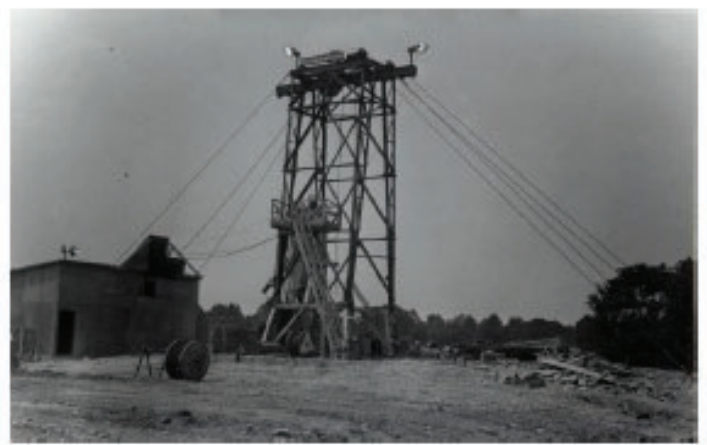
Inland Steel – installation of Coal Hoist – June 1966
