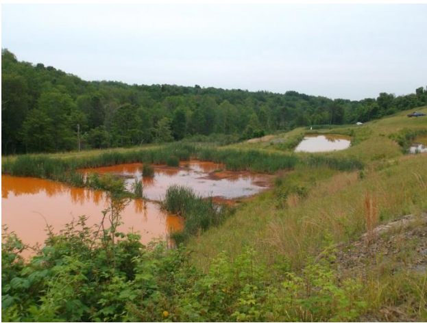
Several of the ponds used in the passive treatment system are shown. The trompe is located at the far end. Photo courtesy Greg Mergenthaler, Carter-Roag Coal Company
