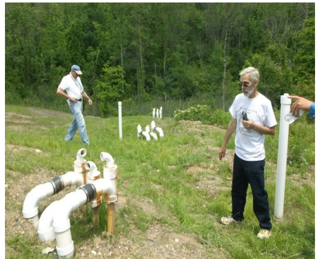
Bruce Leavitt explains the trompe system. Photo courtesy Greg Mergenthaler, Carter-Roag Coal Company
